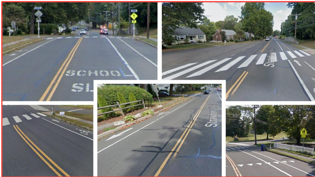
Strawberry Hill Avenue Pavement Markings depicting crosswalks, bike lanes, yield markings, and school warning markings
