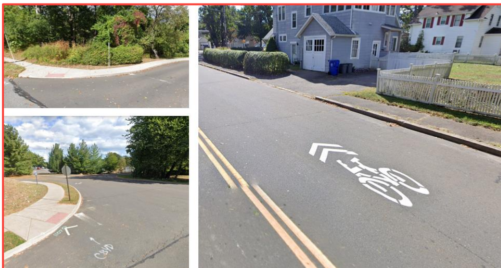
Norden Place Pavement Markings depicting shared bike lanes and crosswalks at both the Northern and Southern Site Driveways
